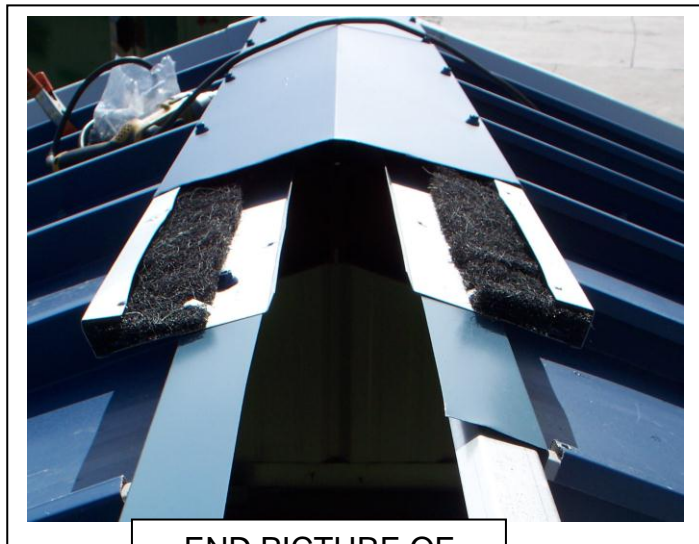
END PICTURE OF PROGRESSIONAL ASSEMBLY
